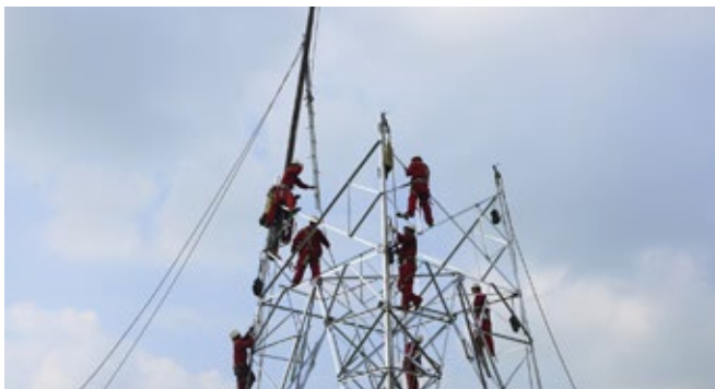
Tower Erection
